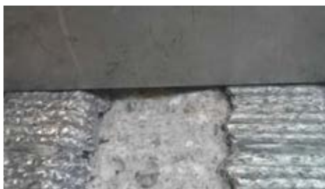
Fig. 4: Uneven concrete removal between two reinforcement rods.
